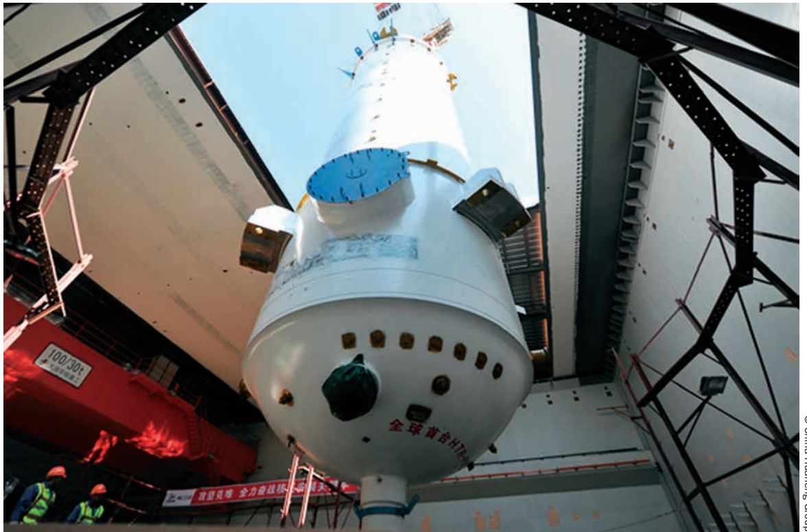
An HTR-PM reactor pressure vessel is lowered into the reactor building.
